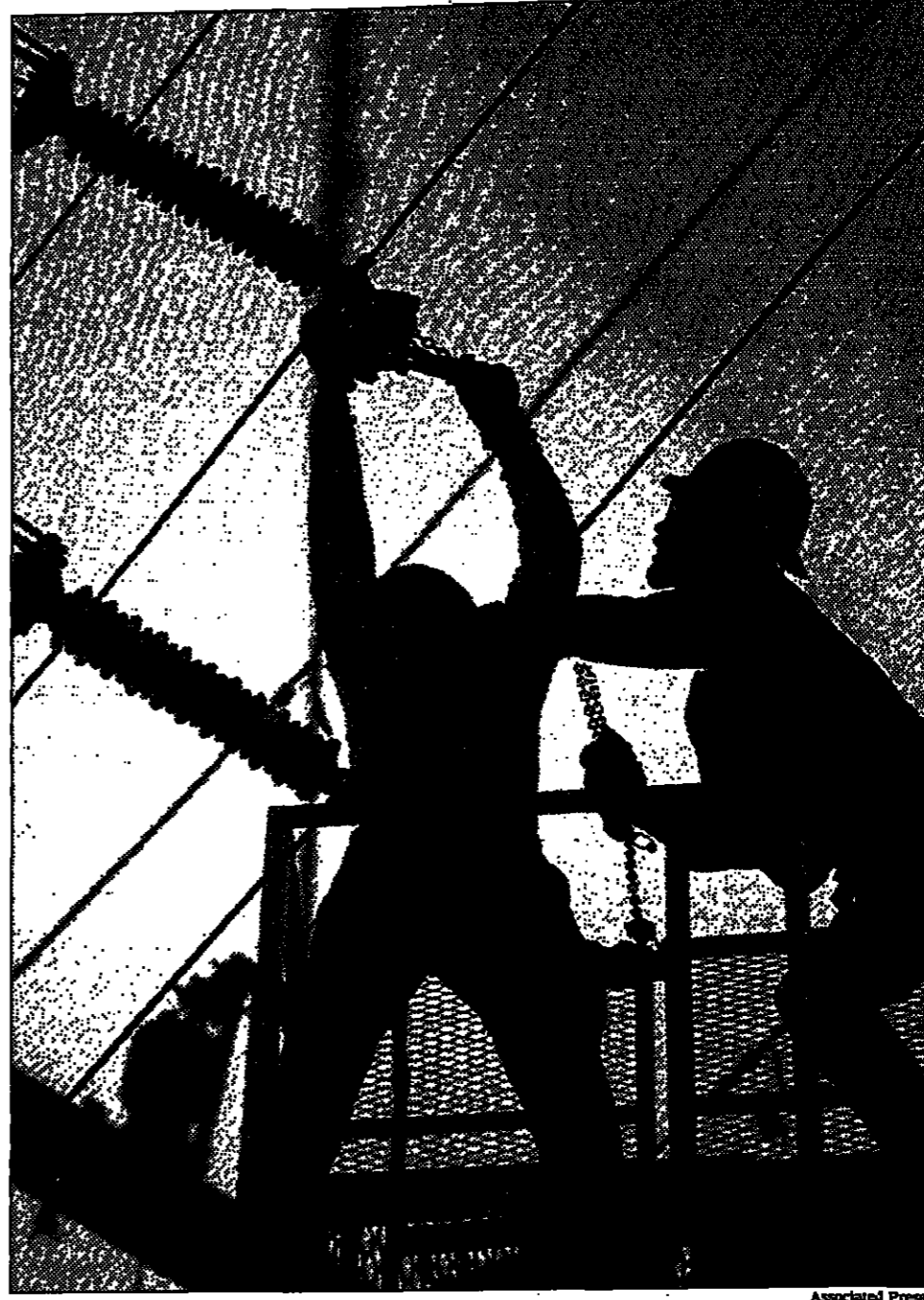
Workers repairing lines in California, a state set to deregulate electric monopolies.
